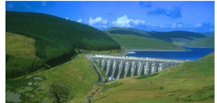
Figure 1. Nant-y-Moch dam, part of a 55 MW hydroelectric scheme in Wales. Photo © Dave Newbould, www.origins-photography.co.uk
