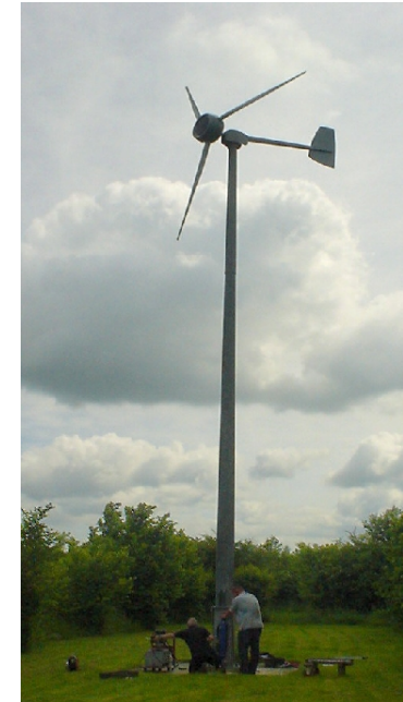
Figure 1. A 5.5 m diameter Iskra 5-kW mini-turbine having its annual check-up. This turbine, located in Hertfordshire (not the windiest of locations in Britain), mounted at a height of 12 m, has an average output of 11 kWh per day.
