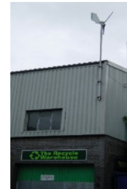
Figure 2. The average power generated by this Ampair 600-W micro-turbine in Leamington Spa is 0.037 kWh per day (1.5 W). For comparison, the average British person's share of electricity consumption is 17 kWh per day.
