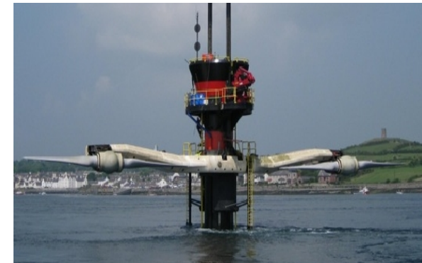
Figure 1. Seagen (Strangford Lough), the first grid-connected tidal stream device in the UK, with capacity of 1.2 MW. Photo by Dr. I.J. Stevenson.
